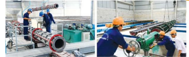
Ráp khuôn/ Framework installation
